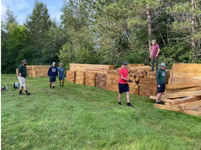
Crews moving eastern larch timbers to deflector structure sites.
