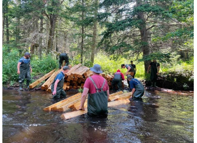
Crews moving eastern larch timbers to deflector structure sites.
