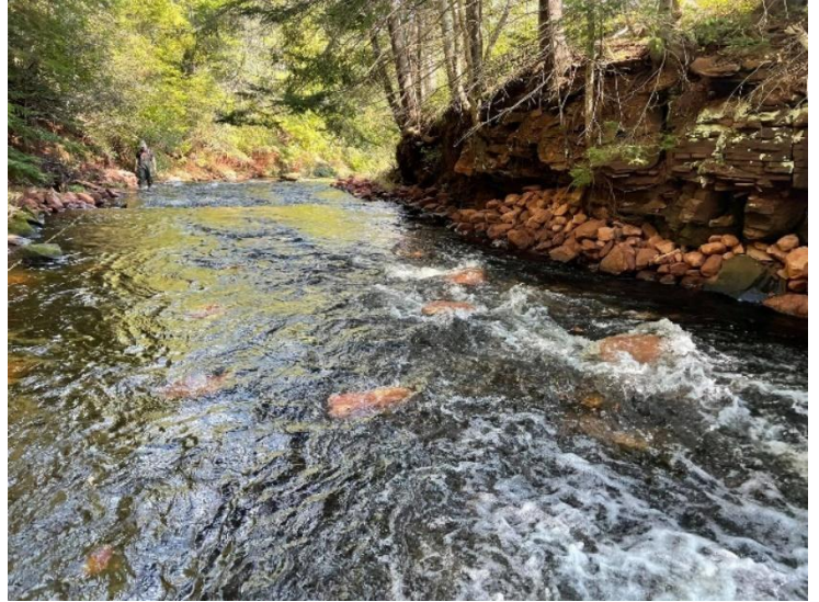
New bank protection consisting of the rock toe, hay bales and alder brush matting. Large rock in the center of the channel for fish resting areas.
