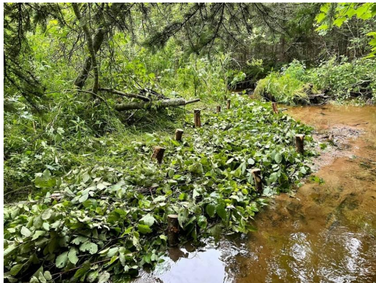
Heavy sediment load along the South Branch of the Morell River along with newly constructed brush mats.
