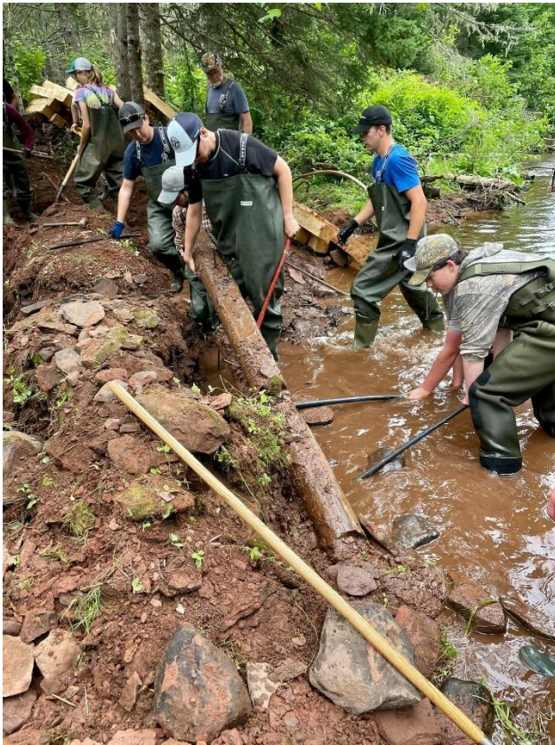
Tearing out the old deflector. New deflector filled in with river rock.
