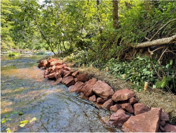
New bank protection consisting of the rock toe, hay bales and alder brush matting. Large rock in the center of the channel for fish resting areas.
