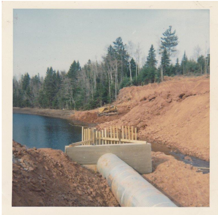
New bypass construction to create fish passage at Leard's Pond. Photo provided by Linda Campbell.
