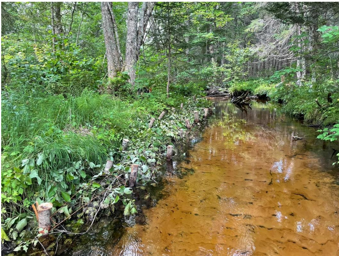
A brush mat built along the south branch of the Morell River to collect excess sediment.
