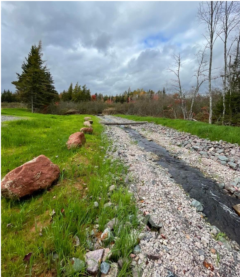
Nature-like fishway constructed by Ducks Unlimited Canada at McKenna's Pond (2021).
