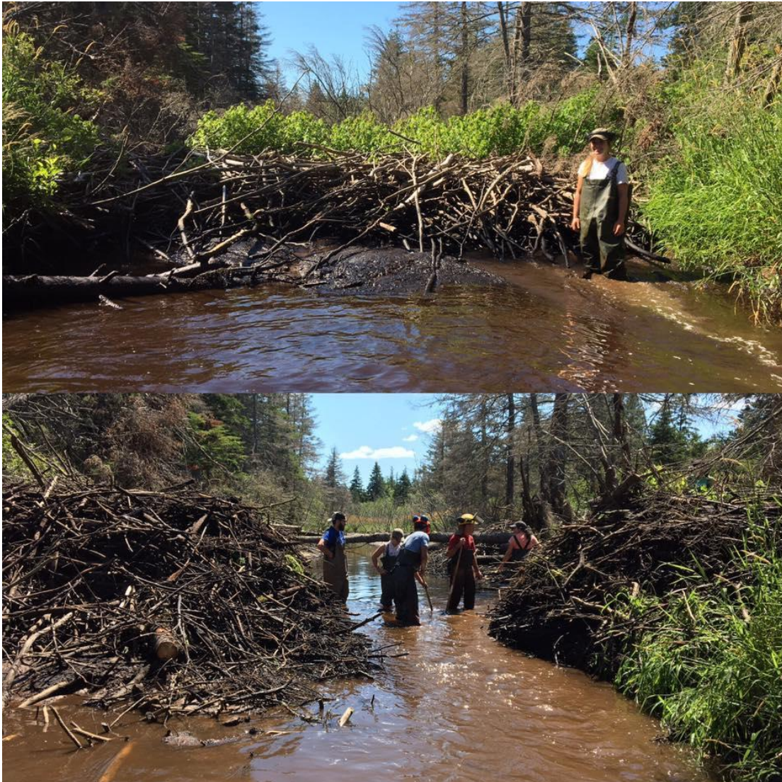
An inactive beaver dam removed to re-establish fish passage.
